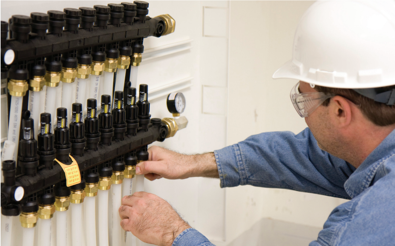
Figure 4-3: Uponor engineered polymer (EP) manifold
