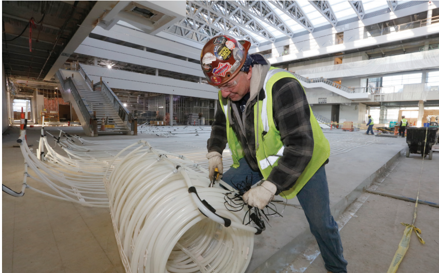
Figure 5-5: Uponor Radiant Rollout Mat
