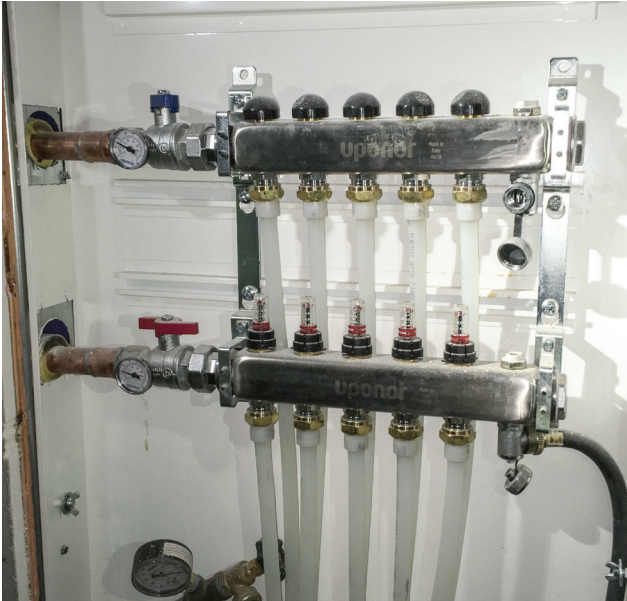
Figure 4-1: Uponor stainless-steel manifold
