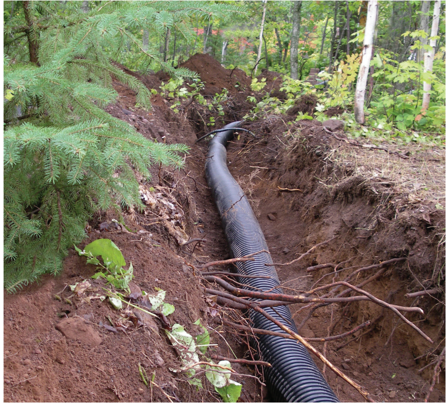
Figure 5-7: Uponor Ecoflex pre-insulated pipe
