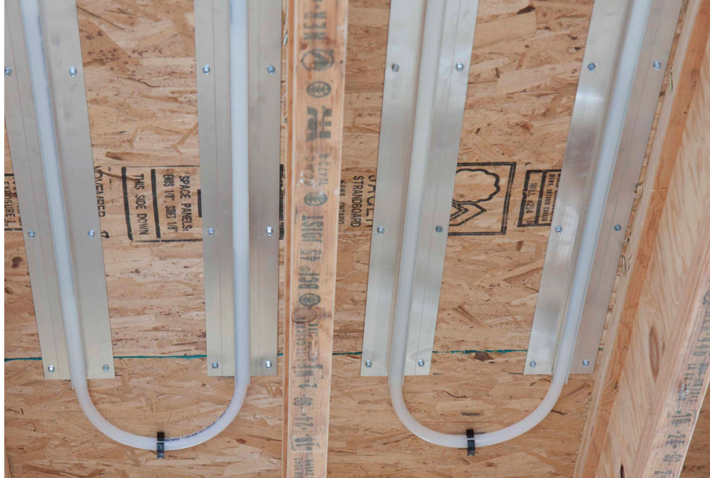
Figure 7-4: Joist Trak aluminum heat transfer plates
