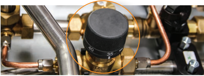
Figure 3-4: Temperature bypass valve
