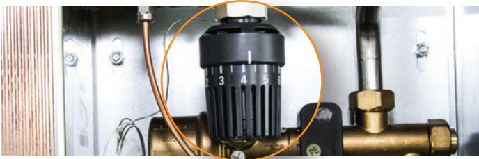
Figure 3-5: DHW controller
