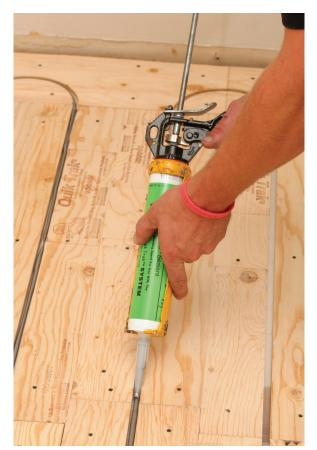
Figure 26: Apply a thin, <sup>1</sup>/<sub>8</sub>" bead of 100% silicone sealant to the entire length of the Quik Trak straight panel grooves. Do not apply the silicone sealant to the return panel grooves.
