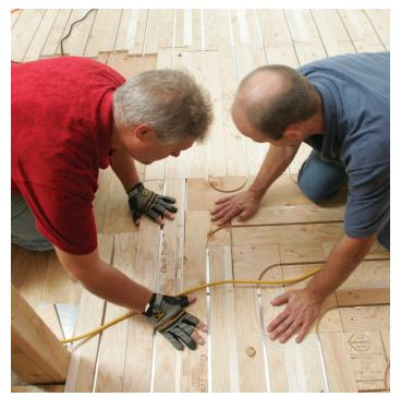
Figure 3: Installing Quik Trak straight panels
