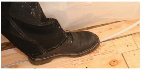
Figure 27: Use hard-soled boots or shoes to walk the piping into the panel groove.
