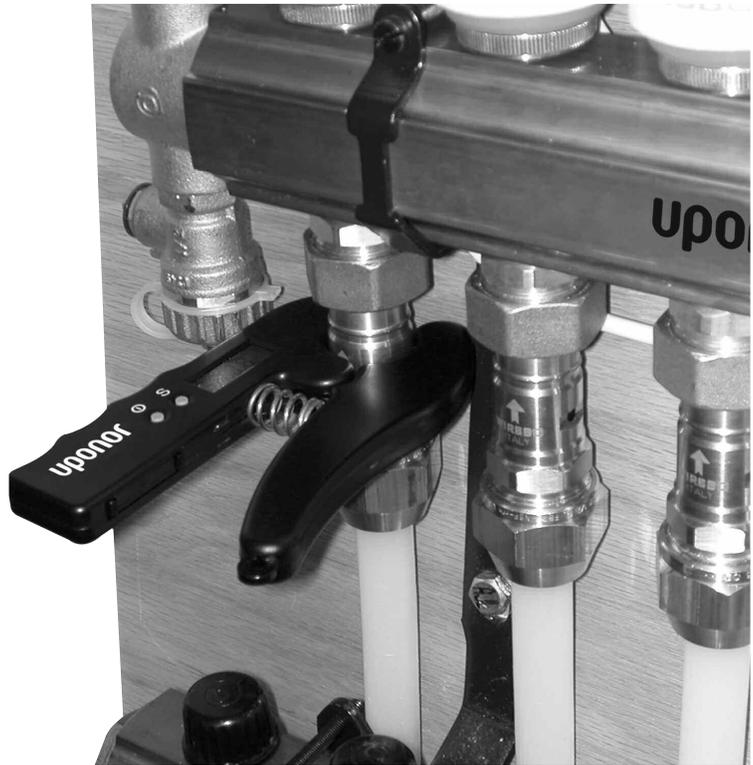
Figure 3: FlowMaster Jr. Attached to Flow Meter Nipple
