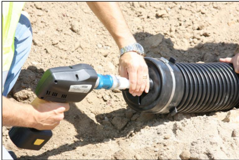
The ASTM Ecoflex line uses Uponor’s durable ProPEX® expansion fittings, featured above, or WIPEX™ dezincification-resistant (DZR) brass compression fittings.
