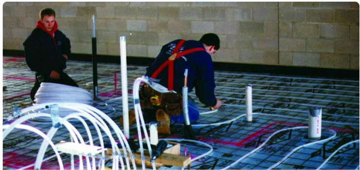
Pat McNamee's own employees installed the Uponor radiant floor heating system in the offices and warehouse of the new facility.
