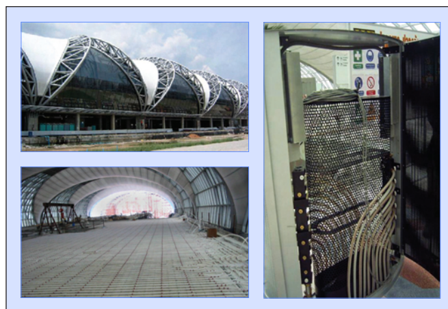
Figure 5: Installation of floor cooling with manifolds in the displacement diffusers at the new Bangkok airport.
