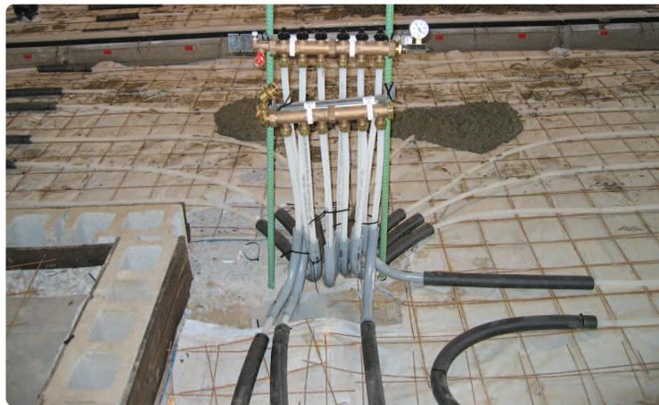
Using Uponor PEX tubing speeds installation because the flexible tubing bends, eliminating the need for extra fittings and joints.
