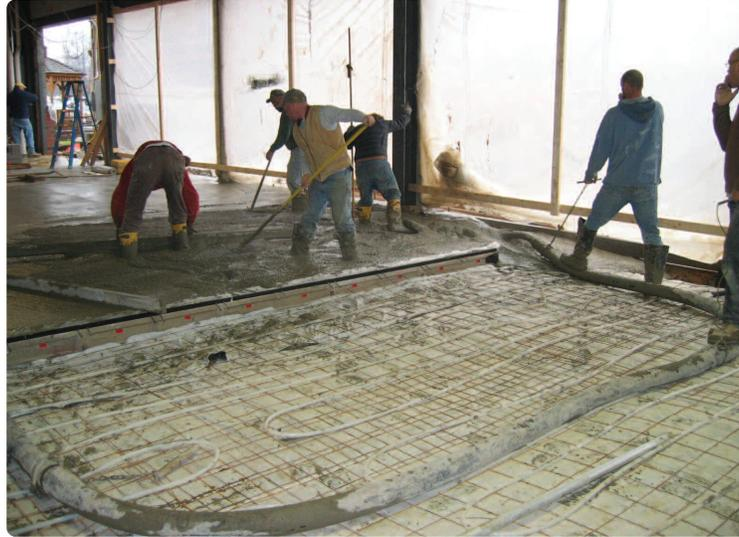
Installers fasten Wirsbo hePEX™ plus to wire mesh and then pour concrete over the tubing to create the warm slab.
