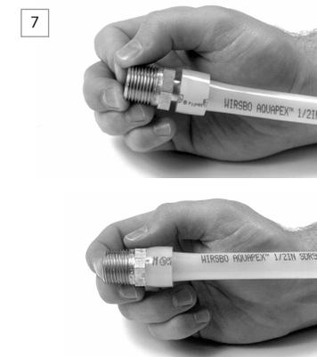
7. Immediately remove the ProPEX expander tool. As you slide the tubing over the fitting, you should feel some resistance. If the tubing reaches the shoulder of the fitting without any resistance, the tubing may be over-expanded and may require additional time to fully shrink over the fitting. The tubing and ProPEX Ring should seat against the shoulder of the fitting for a proper connection.
