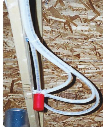
The sprinklers in the Uponor fire protection system offer reliable protection and will only activate when the surrounding temperature reaches 155°F.
