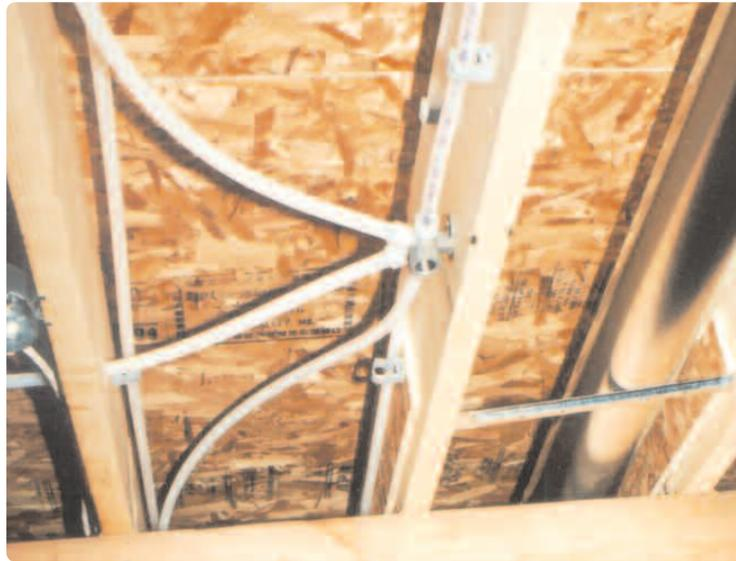
Uponor's residential fire protection system is completely integrated with the cold-water plumbing system, providing the only non-stagnant multi-purpose system available.
