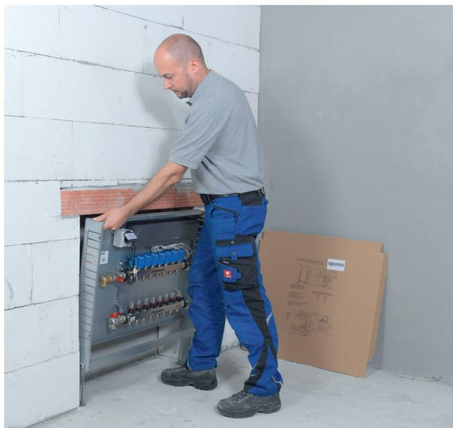
The comfort ports are already quipped with two spirit levels built into the cabinets for easy leveling without additional tools for horizontal and vertical leveling.
