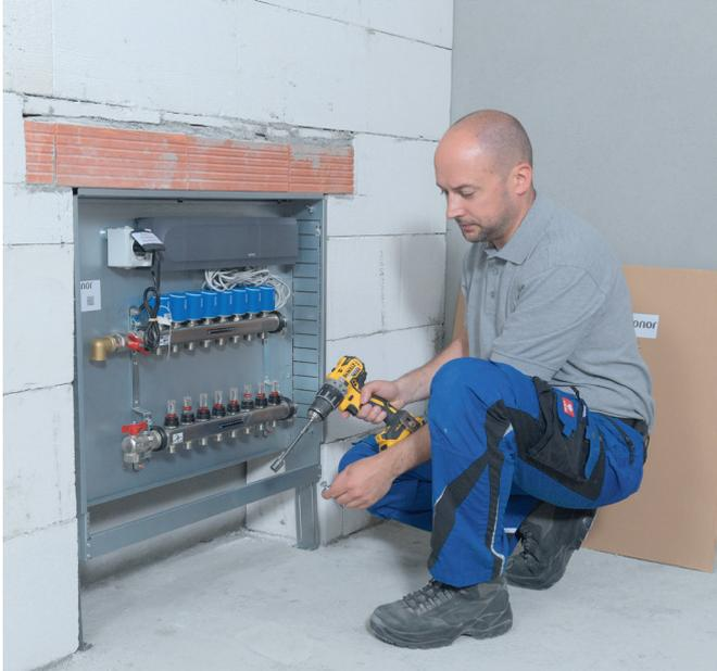
During work interruption at the Comfort Port as well as during plastering and screed work the built-in components should be protected against damage and contamination with delivered protective cover.
