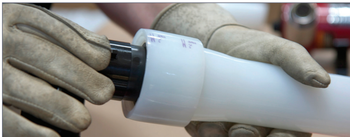
Figure 2-26: Insert fitting
