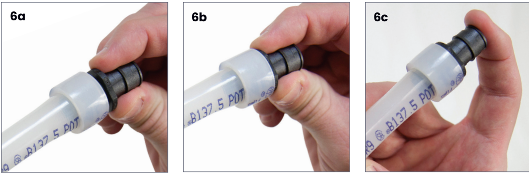
Figure 2-5: Inserting ProPEX fitting into 1/2" Uponor PEX piping
