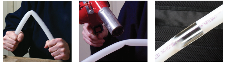
Figure 6-1: Reforming kinked piping
