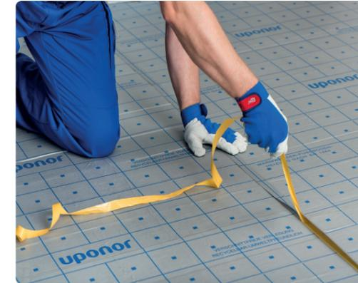
Self-adhesive strip along the panel for quick butt panels connection - just remove the safety tape and connect the panels.
