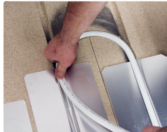
Just a few components for a fast installation: panel, turning plate, multi heat emission plate extra and heating pipe
