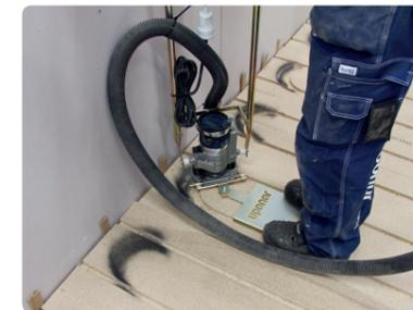
Use the Uponor milling machine to make grooves or use specially made turning plates.
