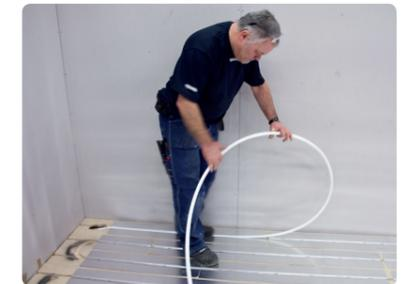
The pipes are positioned and fixed in place in the heat emission plates.
