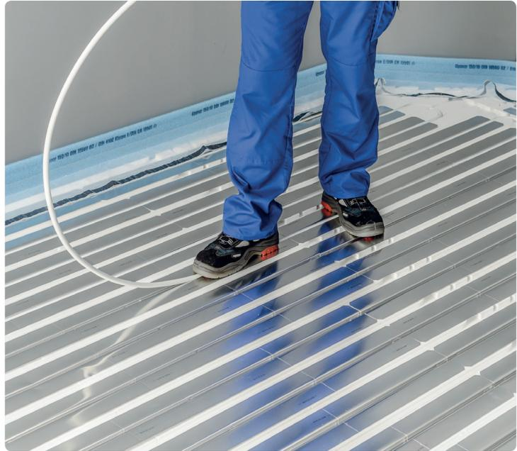
The integral pipe guide channels in the Siccus mounting sheet hold the heat conducting plates and heating pipes
