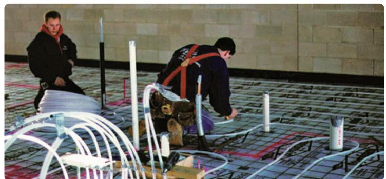
Employees at Pat's Heating & Air Conditioning, shown installing the Uponor radiant floor heating system in their building in 1997. The company now does up to 15 radiant installs annually.
