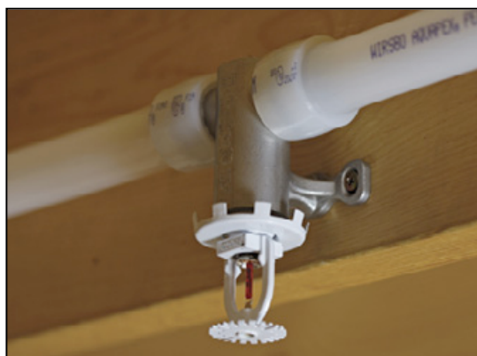
The new AQUASAFE Looped Residential Fire Safety System employs two-port sprinkler fittings with 3/4" and 1" Wirsbo AQUAPEX.
