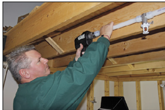
The new multi-purpose AQUASAFE Looped Residential Fire Safety System uses the same Wirsbo AQUAPEX tubing that provides potable cold water to the plumbing fixtures in a home.
